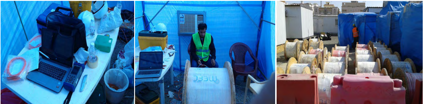
Fiber Optic Cable Drum Test (SECo Jeddah)
