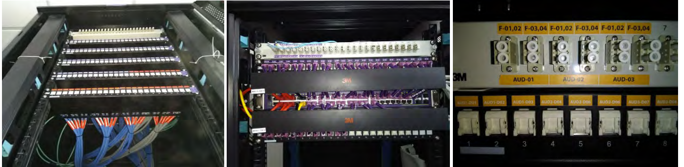
VOX Cinema West Avenue Dammam (Data Center)
