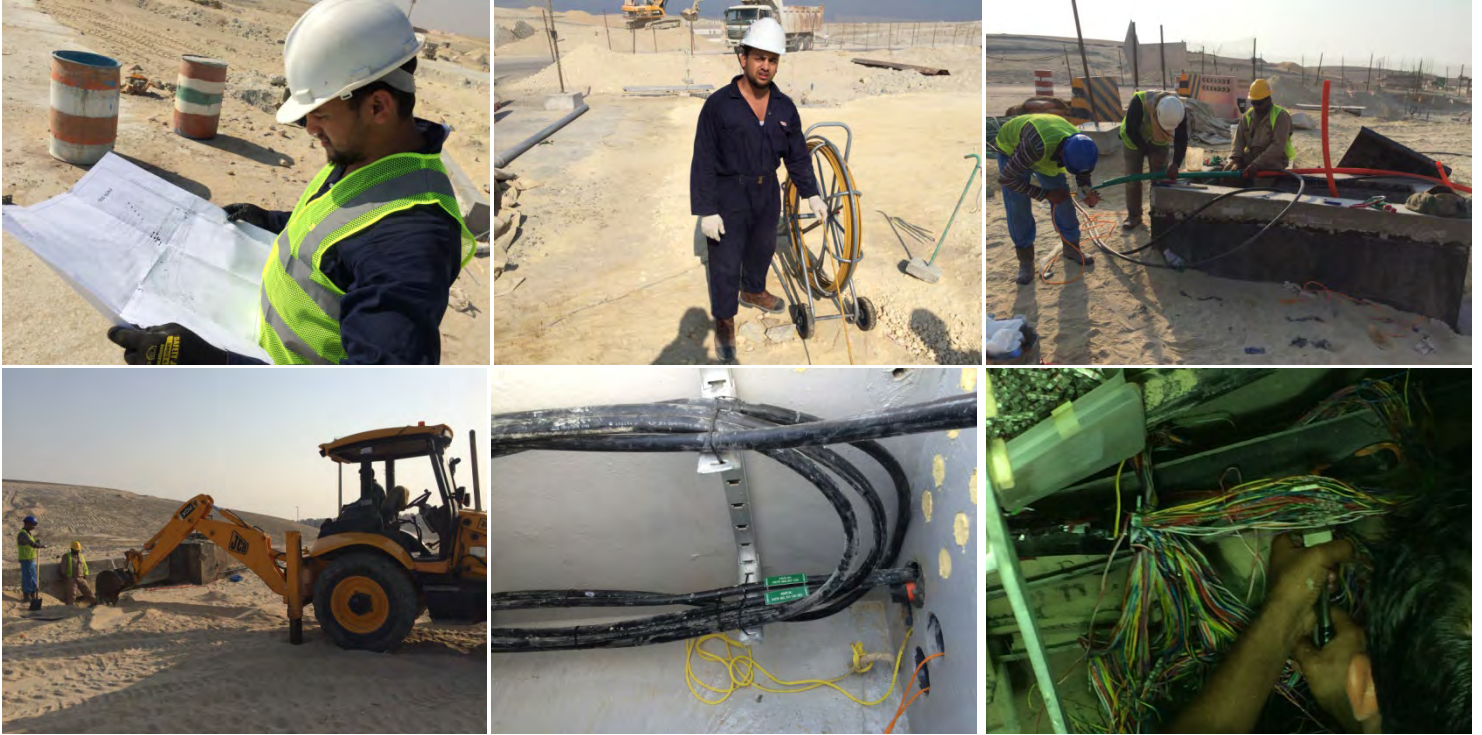
Site Work at Jubail FANATEER Beach Re rooting STC Copper Line
