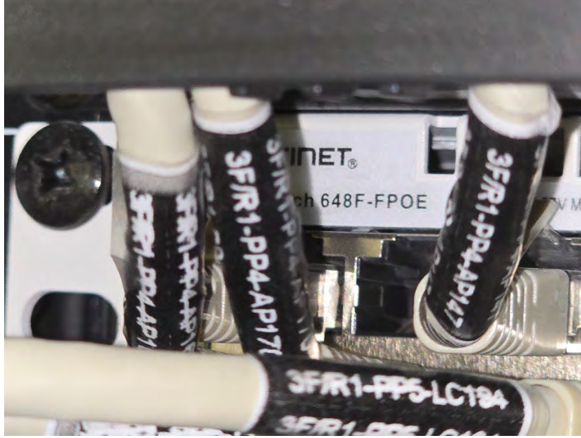
TAHAKOM HEAD OFFICE Riyadh (UTP Patch Cord Labelling)
